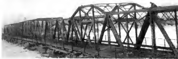
New Steel Bridge completed March 9th.
